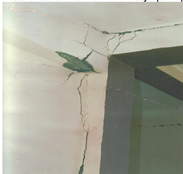
Photo 1 : Fissuration du mur Ain El Hadjel. [C T C]
