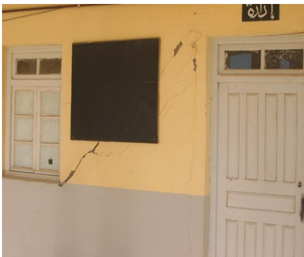
Photo 1 : Fissuration du mur Ain El Hadjel. [C T C]
